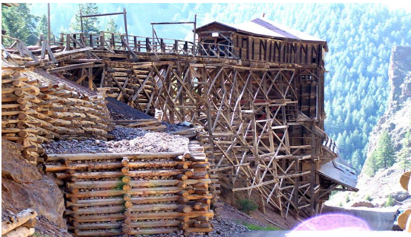
Commodore ore house and chutes coloradohikes.com
